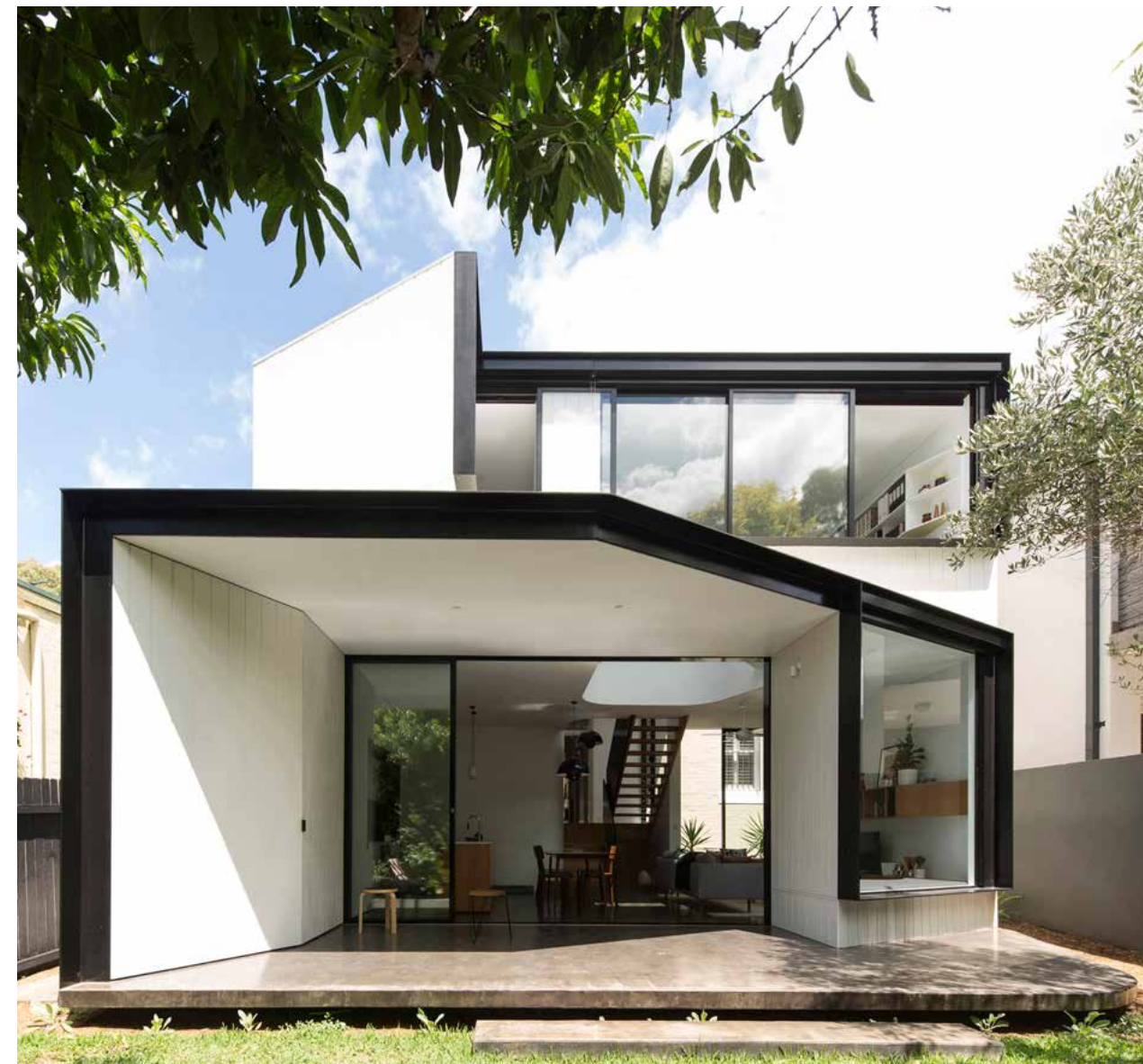
The new rear extension, finished in lightweight Shadowclad ply, is crisply monochromatic. opposite page top left The glazed link between the old house and the new extension accommodates circulation areas. right From the upstairs study area a semicircular cut-away section, as well as multiple windows and the open-riser stair, allow visual connections in all directions. bottom right The new living area features built-in joinery along one wall, including a daybed angled to catch the north-eastern sun.
